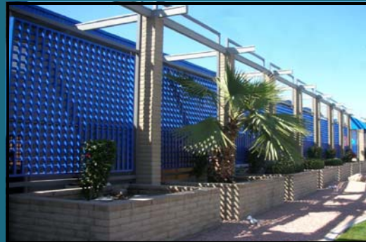
150 + Units located in Central Phoenix Built in 1961, Takeover February 2009
